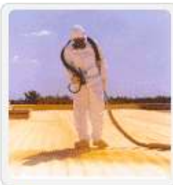
▲ Spray Heat Insulation
